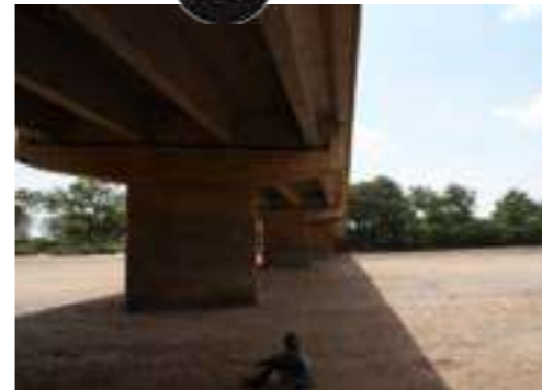
Boy sits under a Tarach bridge in Kakuma Town
